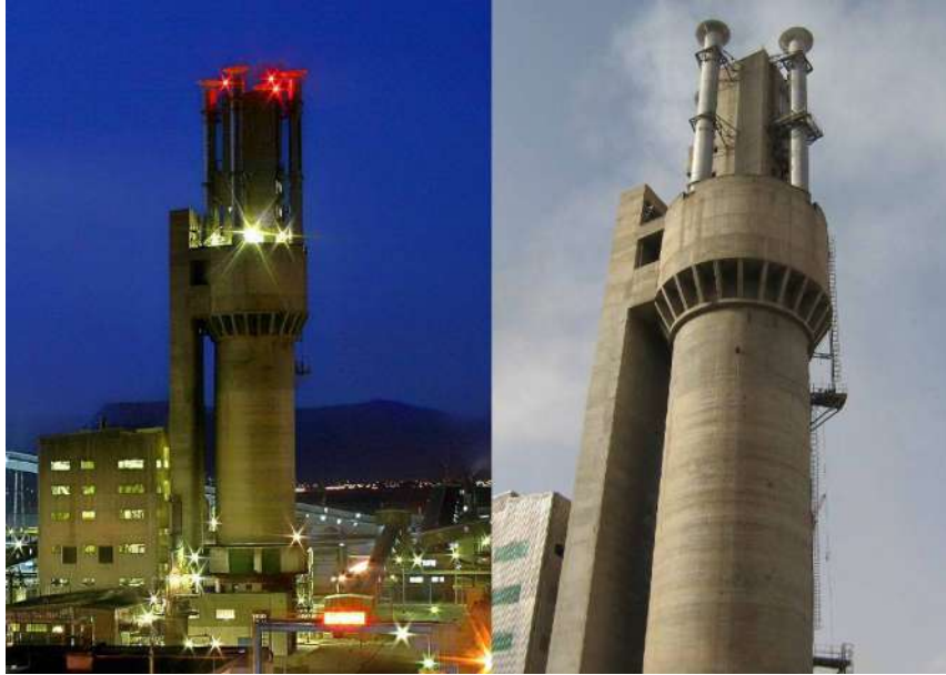
Fig. 1 Ammonium Nitrate periling tower.
